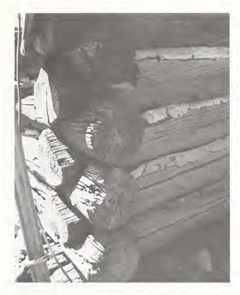
Figure 89. Dovetail corner notching on the Bear Mountain lookout storage shed (original cabin).
